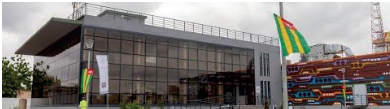
Lomé Data center
